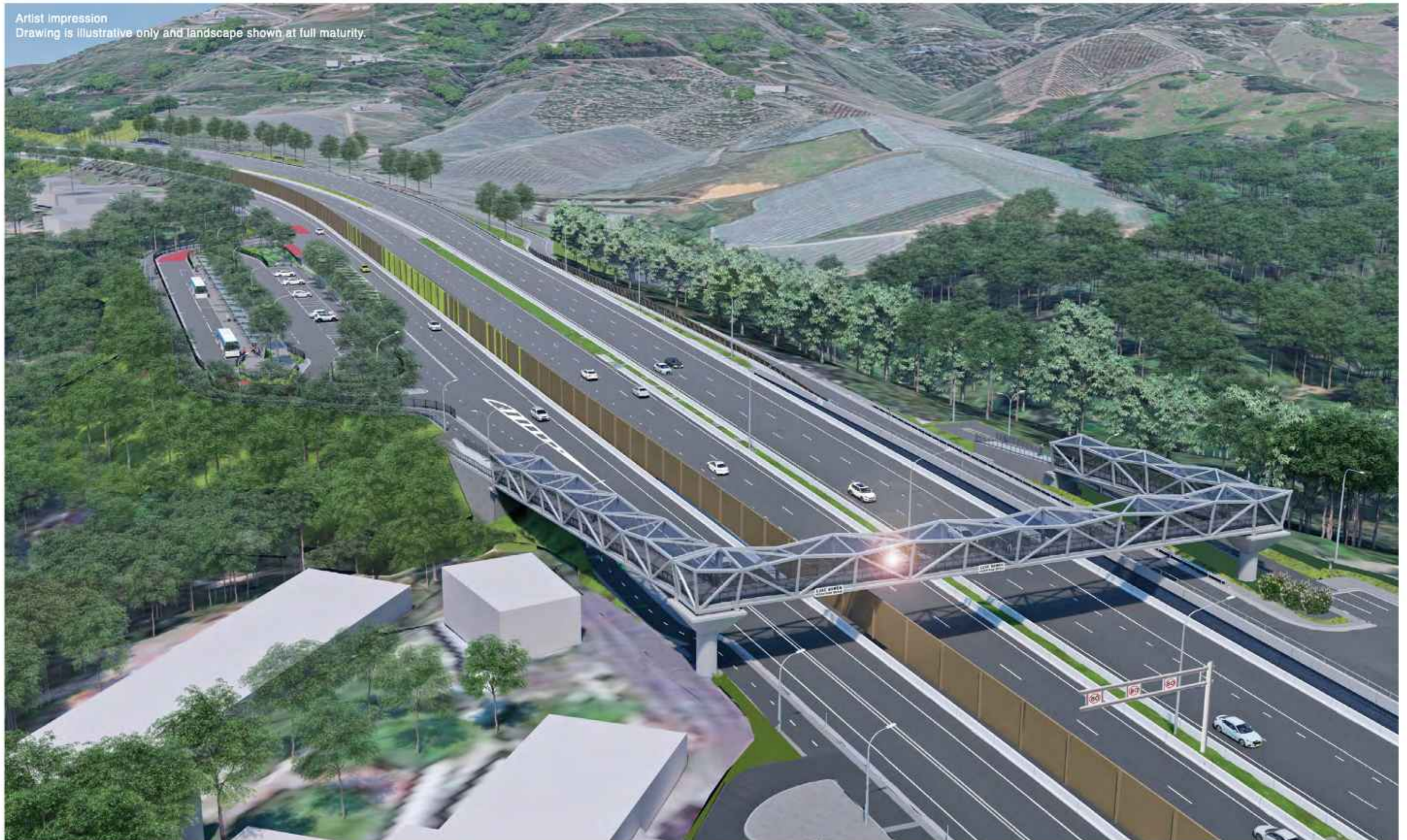
Figure 132: Korora Bus Interchange - aerial view from north east
