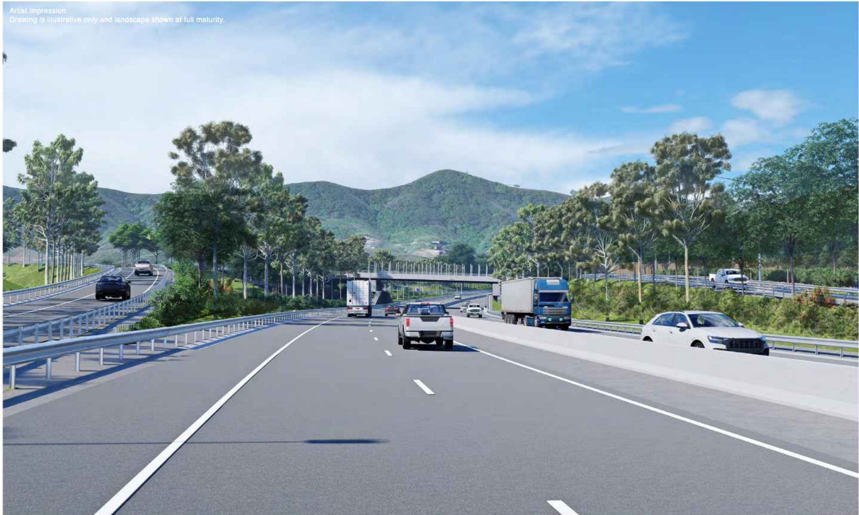
Figure 127: Coramba Road Interchange - view from northbound lanes
