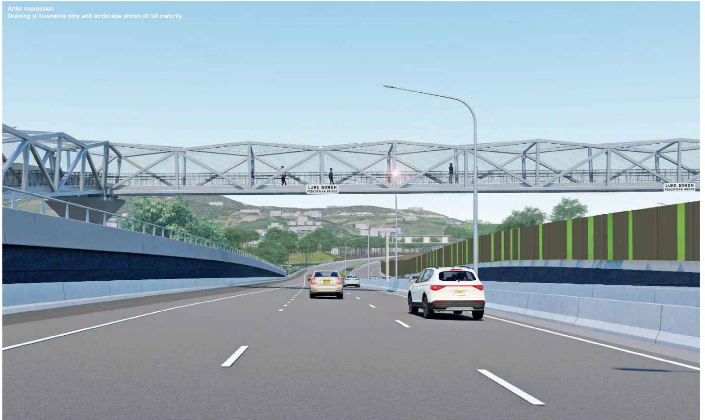
Figure 145: Luke Bowen Pedestrian Bridge (Bridge 24) - looking north
