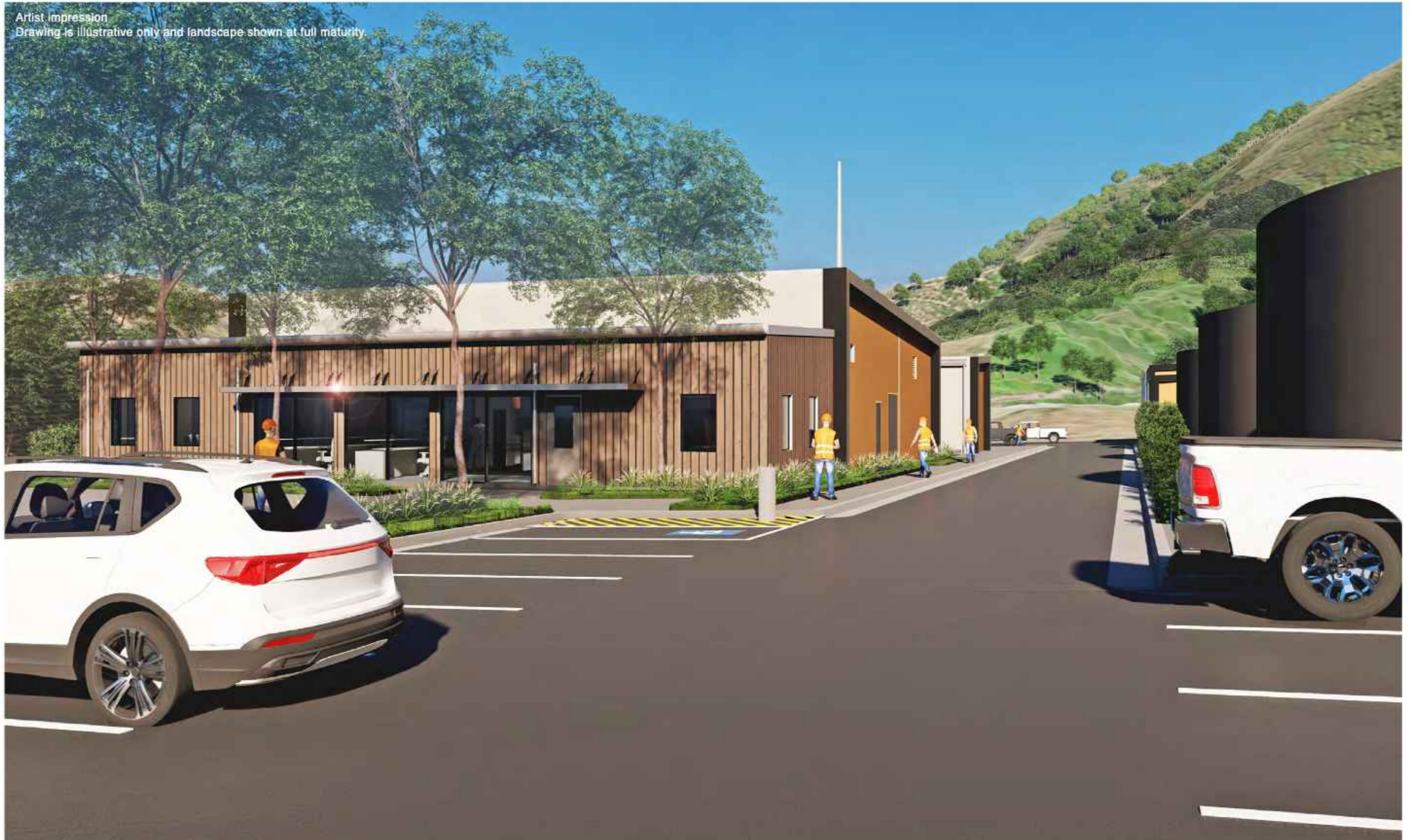
Figure 171: Motorway Operations Maintenance Facility (MOMF) - view from the compound
