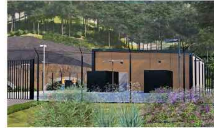
Figure 174: Shephards Lane Tunnel plant and equipment room - building view from front entry
