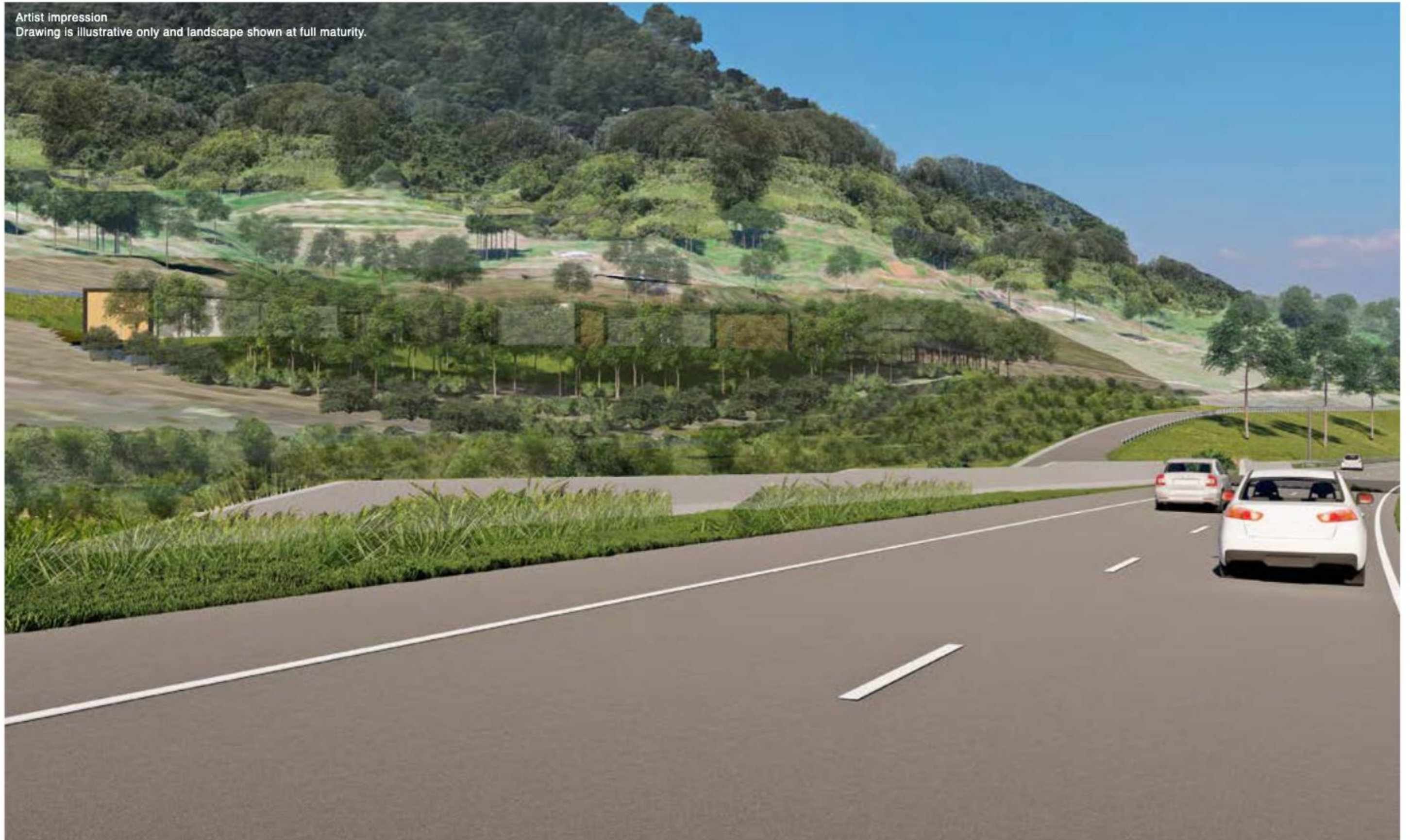
Figure 171: Motorway Operations Maintenance Facility (MOMF) - view northbound lanes
