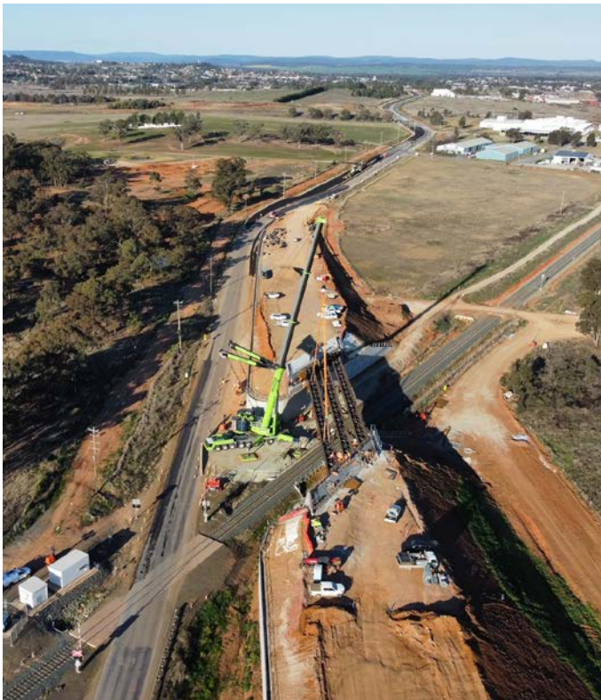
Construction of railway overpass bridge in Parkes
