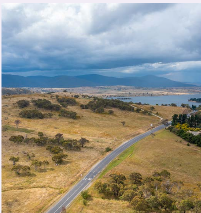
Aerial view of southern connector road into the Snowy Mountains precinct
