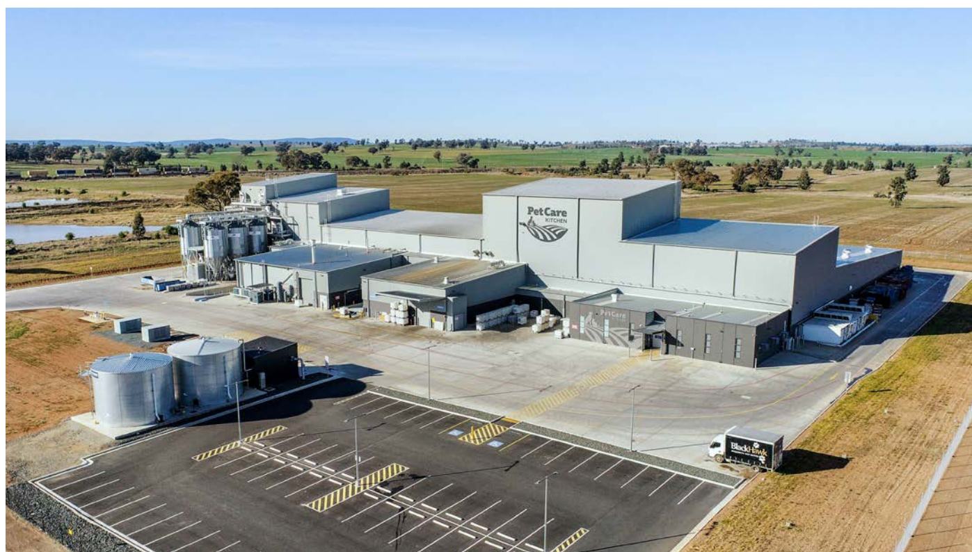
Aerial view of Master Pet facility. Image supplied by Pet Care Kitchen, Parkes NSW.
